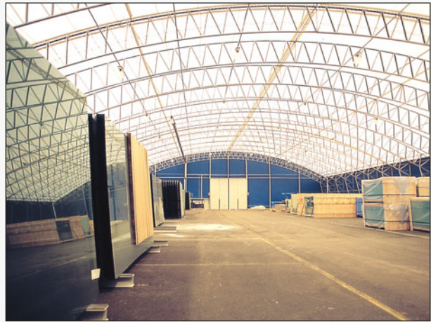
PMH Storage Hall offers maximum floor space with no invasive columns and a translucent roof.
